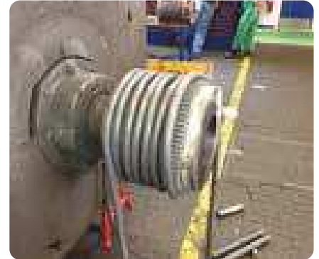
Heating a coupling for dismounting
